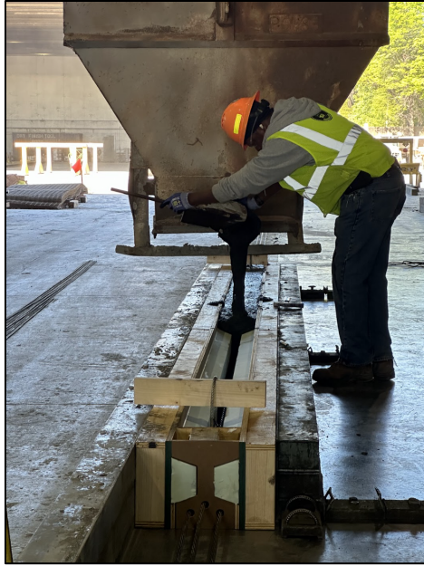
Figure 6: UHPC being poured into formwork.
