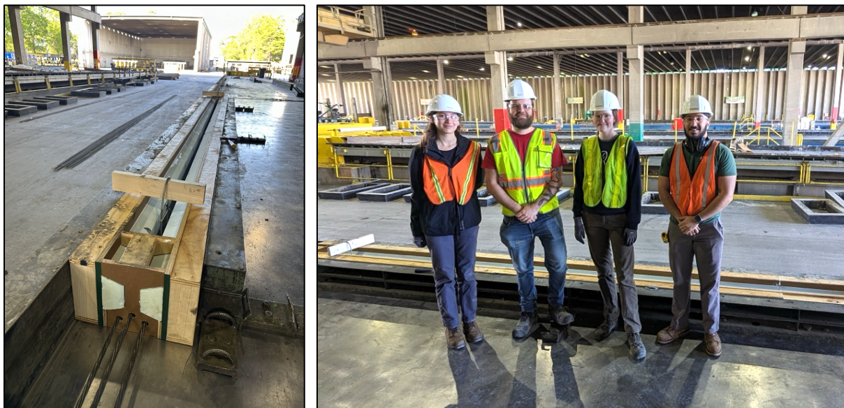
Figure 5: Formwork with Strands (left) and Ready to Cast (right)
